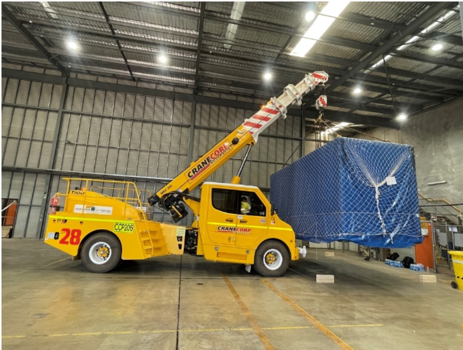
Figure 13 shows a Franna positioning a cabin inside the facility.
