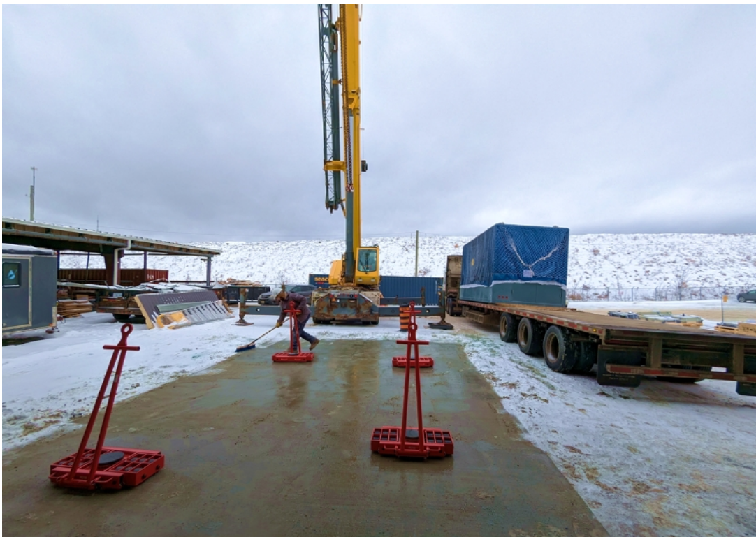
Figure 17 shows the Trolley setup before unloading the cabin off the truck.
