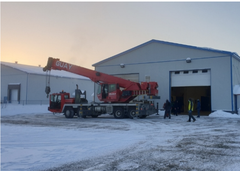
Figure 9 shows an example of the crane positioning for unloading the cabins.
