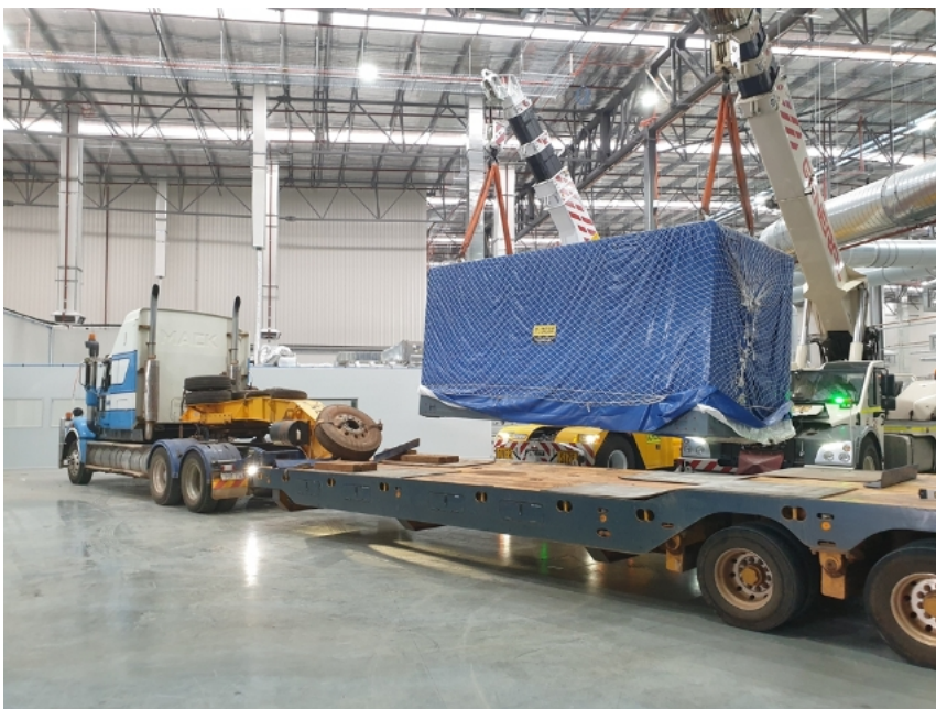
Figure 12 shows two Franna along with the truck unloading Cabin inside the facility.
