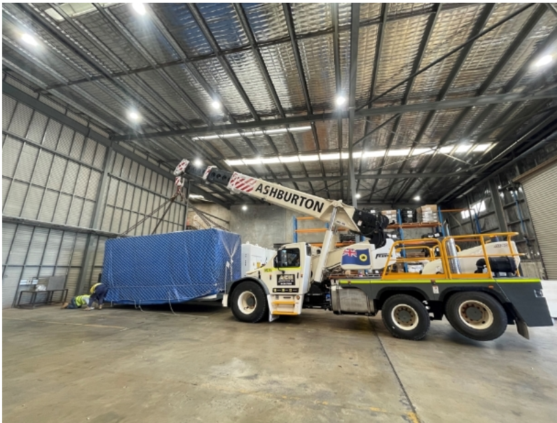
Figure 11 shows 40T Franna positioning the Automation Cabin inside the facility.
